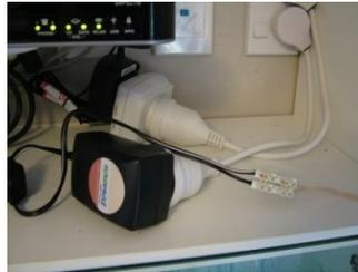
If you require a 240 volt switched outlet to be installed, consult your local electrician. It is recommended that the 240 volt switched outlet and plugin power supply be placed inside a cupboard or somewhere out of sight, with the 12 volt output cable going to the **Unobrain®**.
