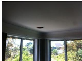
placed in the corner of each room diagonally opposite the doorway 800mm from the window wall and 800mm from the wall at right angles to the window wall. If there is no doorway, a position in the corner of the room should be selected so that the **Univent**® room outlet is towards one end of the window wall using the 800mm by 800mm guideline.
