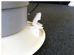
clamps to flip over and pull the surround edge up against the ceiling. After about 3 days, the voltage setting can be set at 9 volts or 7.5 volts to reduce air flow but reset to a higher voltage if the air flow proves insufficient for the reduction of condensation on windows in the winter.
